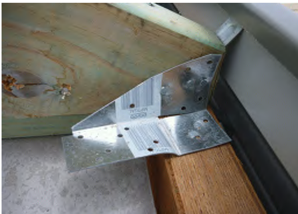
Figure 20. Photograph showing a poorly installed metal connector making the connection between an alfresco beam and rafter
