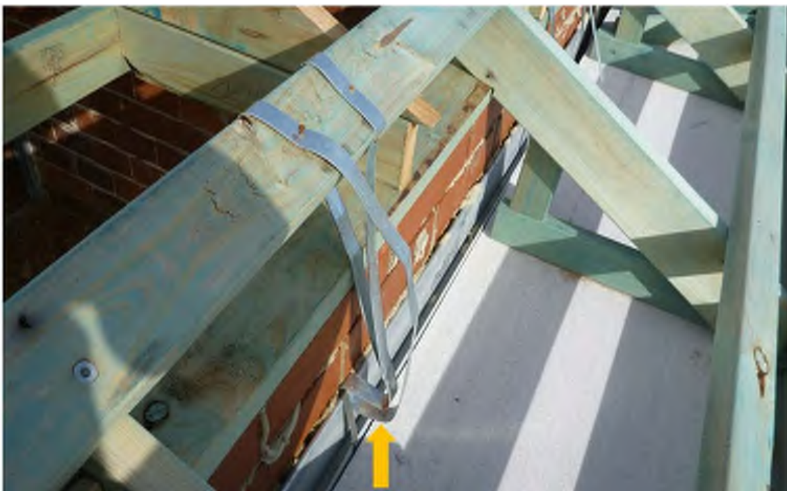
Figure 13. Photograph showing poor installation of tie-down straps
