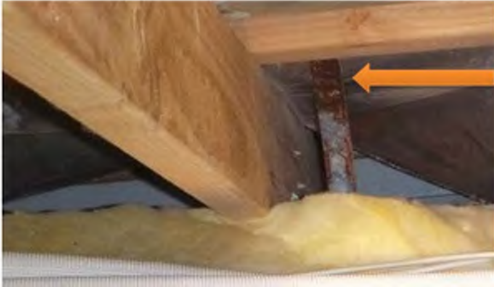
Figure 8. Photograph showing the result of installing a strap without the correct corrosion protection
