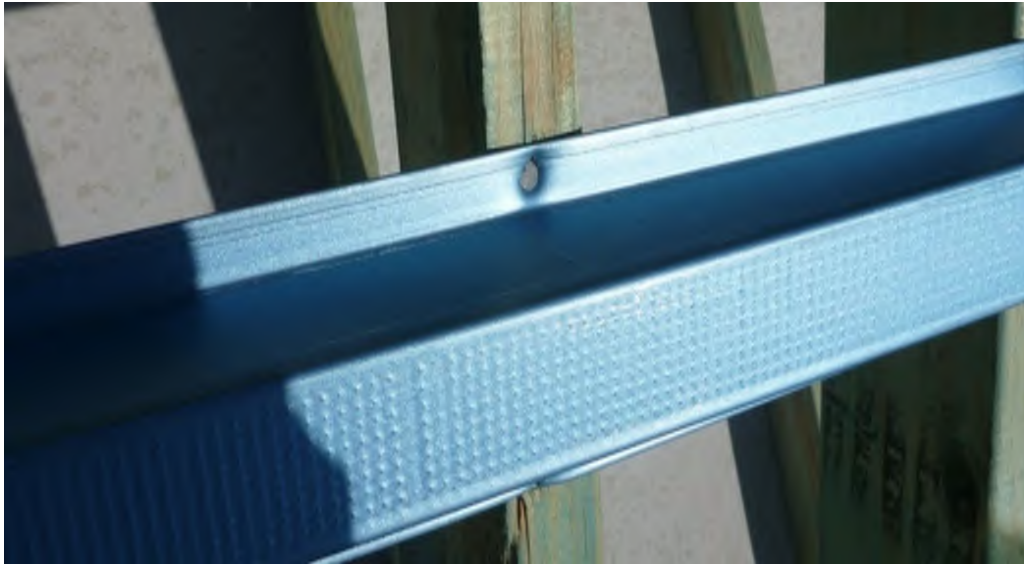
Figure 18. Photograph showing a 75mm x 3.06mm nail over driven when used to fix a metal batten
