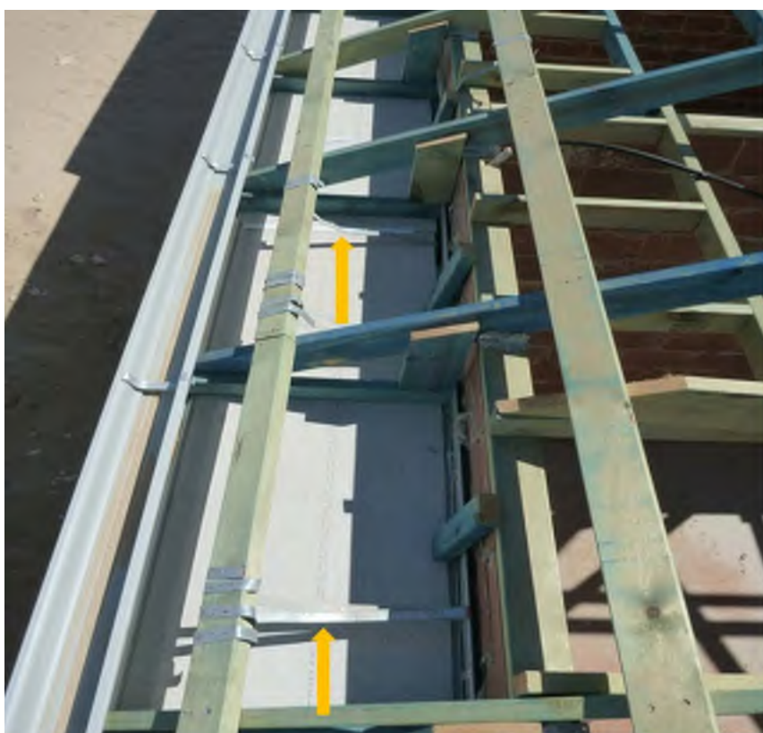
Figure 10. Photograph showing poor tie down strap installation (strap being fixed down the roof line)
