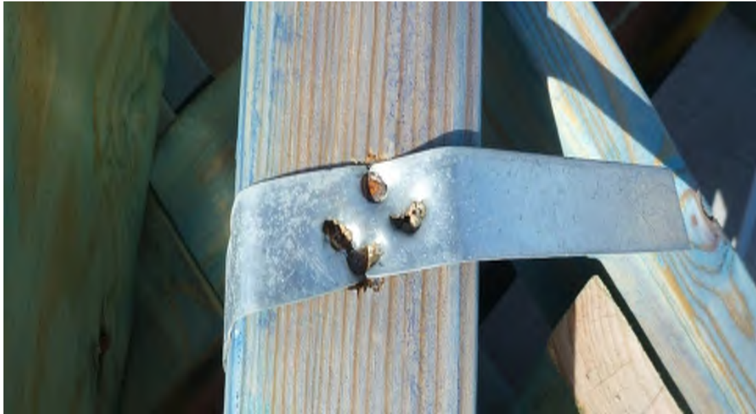
Figure 9. Photograph showing a metal tie-down strap fixed to a batten via the use of machine driven nails. The over-driving of nails has damaged the strap, greatly reducing the connection capacity.
