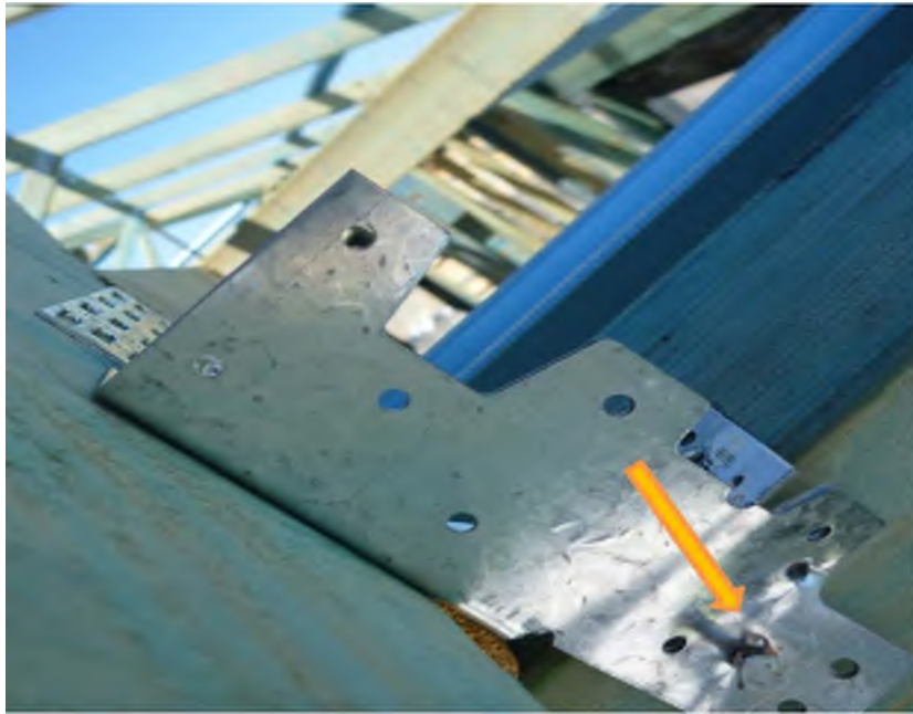
Figure 25. Rafter top plate connection with only one horizontal nail into the top plate tab (Manufacturer recommends 4 nails)
