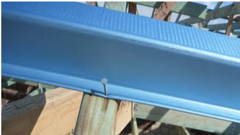
Figure 19. Photograph showing a typical under driven nail fixing a metal batten around this roof
