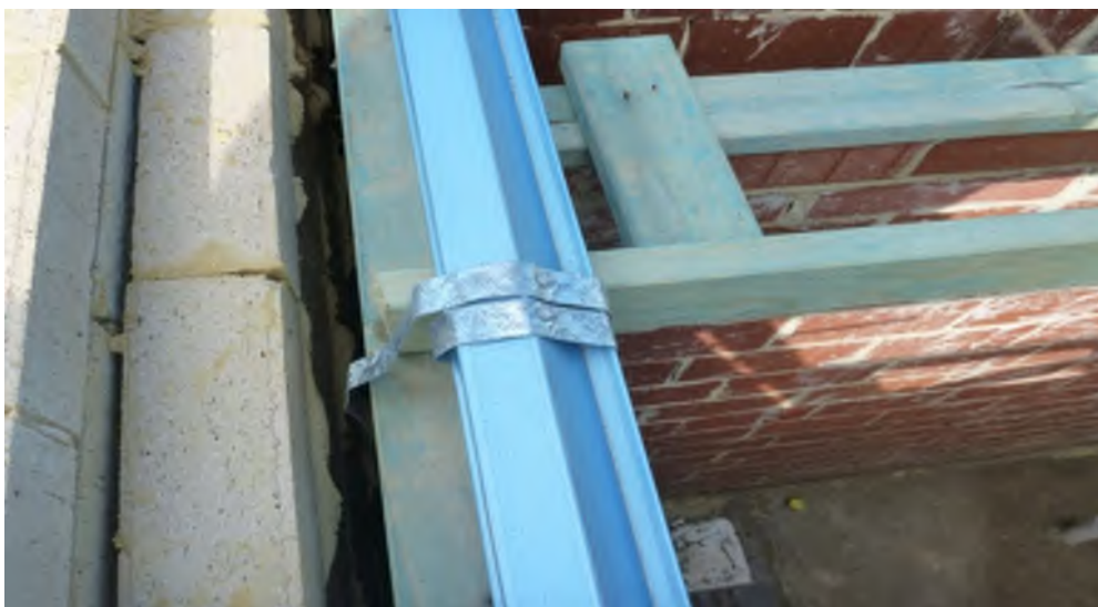
Figure 12. Photograph showing tie-down wrapped around metal batten (Note: the tie down is loose)
