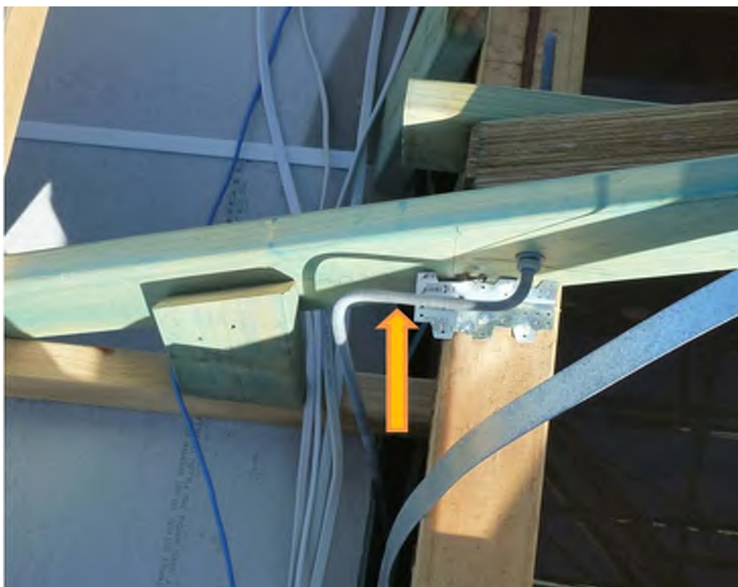
Figure 26. Photograph showing a tie down rod bent to make the connection to the beam
